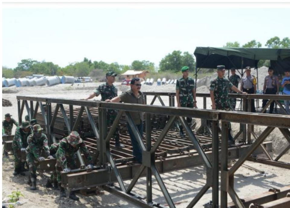
Figure 4-1 : 18 th Engineering Batallion construct a bailey bridge on exercise
