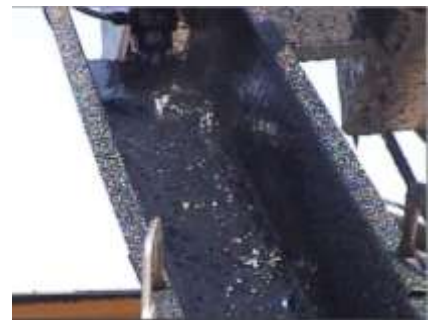
Direct Foaming Asphalt
