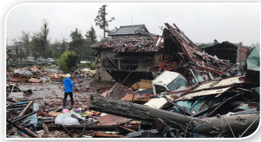
Picture 2.1: Damage caused by super Hagibis typhoon (Retrieved from Thairath Online, 2019)
